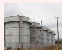
Before installing the fence cover
