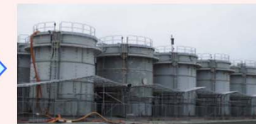
After installing the fence cover
