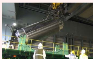
Loading the transportation container onto the trailer
