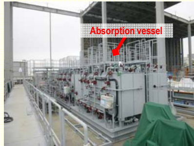
<Installation status of additional multi-nuclide removal equipment>
