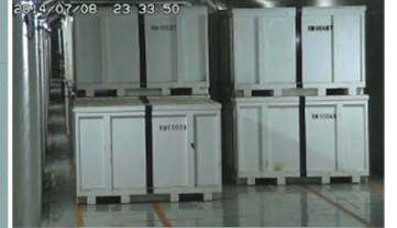
Solid waste storage
