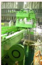
Fuel removal status
