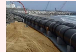
Water pipe installation status (2)
