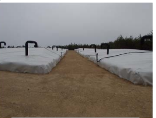
Temporary trimmed trees storage pool
