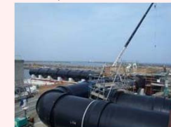
Water pipe installation status (1)
