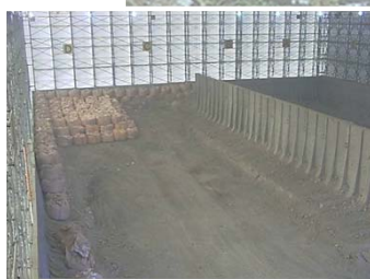
Inside the rubble storage tent
