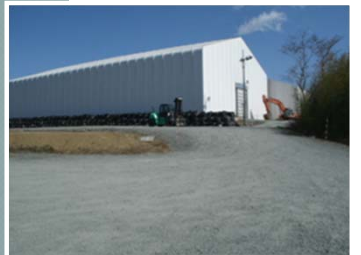
Rubble storage tent
