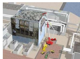
Removal of rubble from the roof of the Reactor Building
