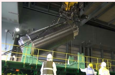
Loading the transportation container onto the trailer
