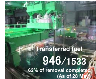
(Fuel removal operation)
