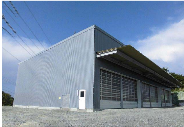
Figure 8: External appearance of the vehicle maintenance site
