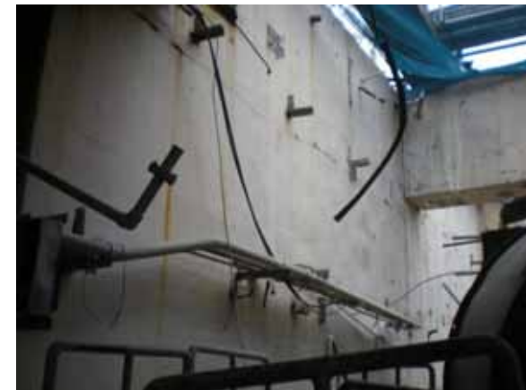
10 Wall on the SFP side (West)
