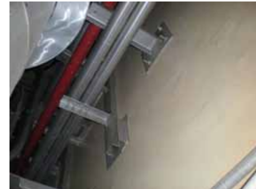
② South wall
