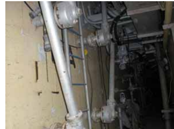
8 Wall on the SFP side (South)
