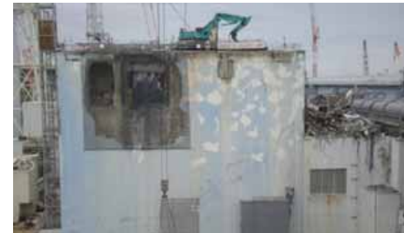
⑥ South wall (Exterior wall)
