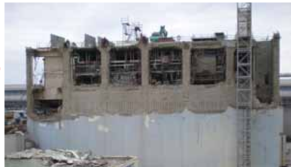
⑤ West wall (Exterior wall)
