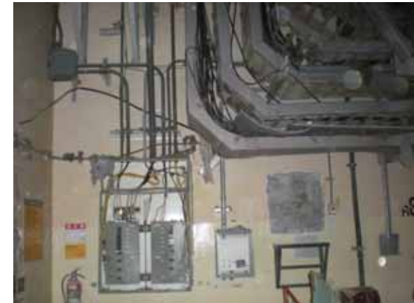
④ West wall (Interior wall)
