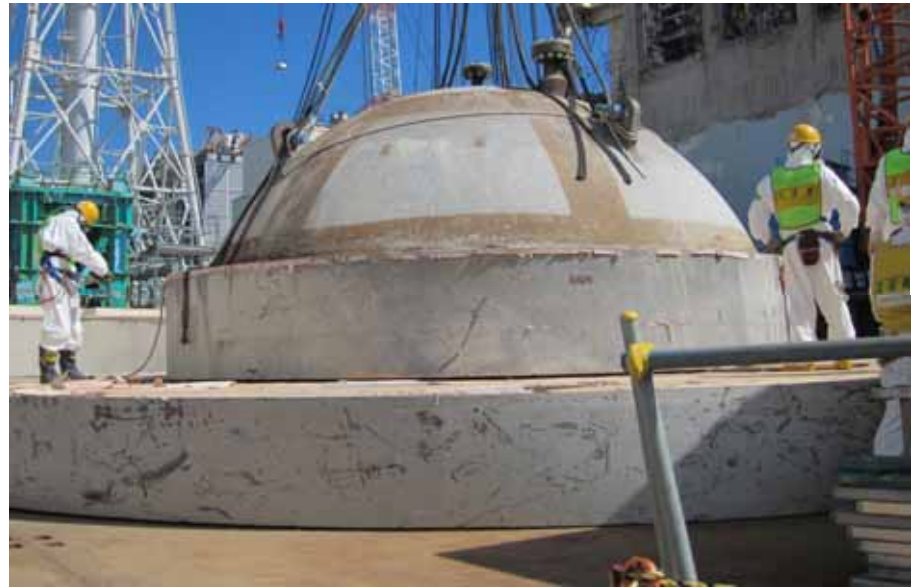
RPV upper lid down on the ground
