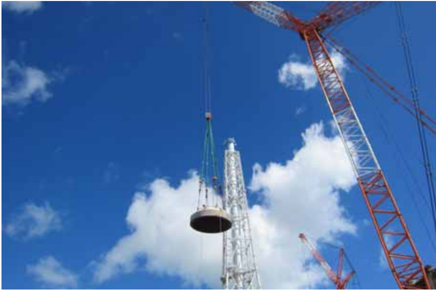
RPV upper lid being lifted up above the operation floor
