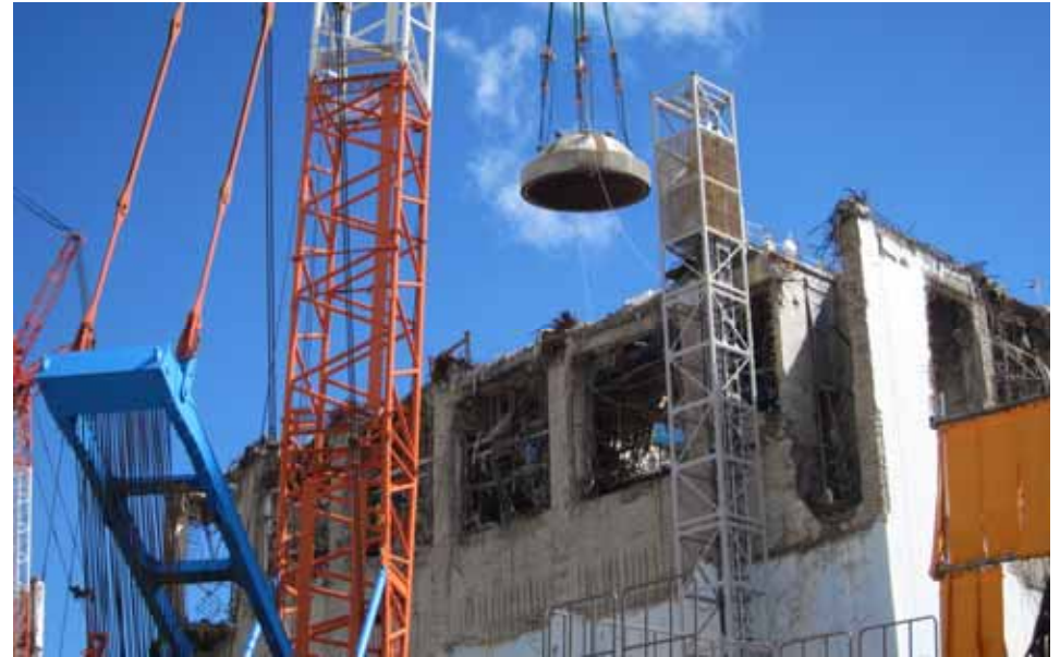
RPV upper lid being lifted up above the operation floor
