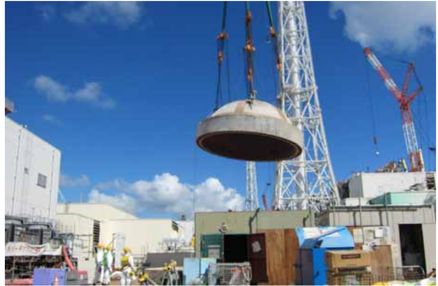
RPV upper lid being lifted down
