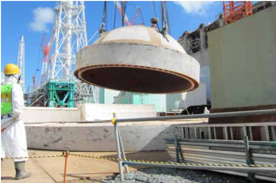
RPV upper lid being lifted down
