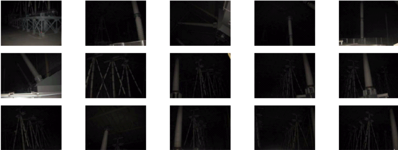
(18)Unit 5 and 6 Ultraigh Voltage Switchyard Area (Inside) [Date the photos were taken (gathered): March 22, 2011] Photos taken by a TEPCO employee 15/600 photos
