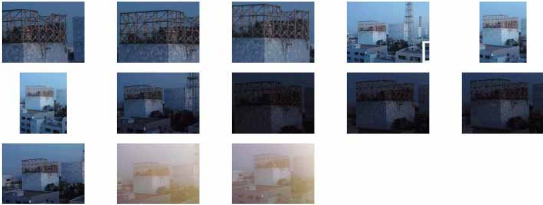
(7) Appearance of Unit 1 after the explosion [Date the photos were taken (gathered): March 12, 2011] Photos taken by a TEPCO employee 13/600
