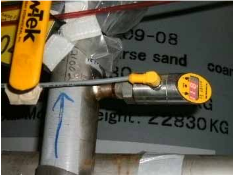
Before replacement (PIT100B)
