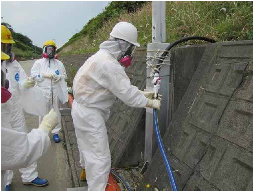
Temporary hose installation (Outside)
