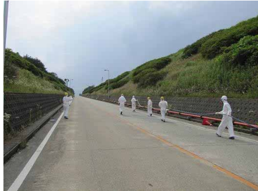
Temporary hose installation (Outside)
