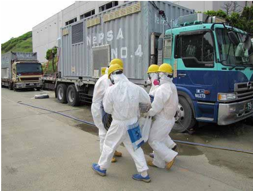
Temporary hose installation (Outside)
