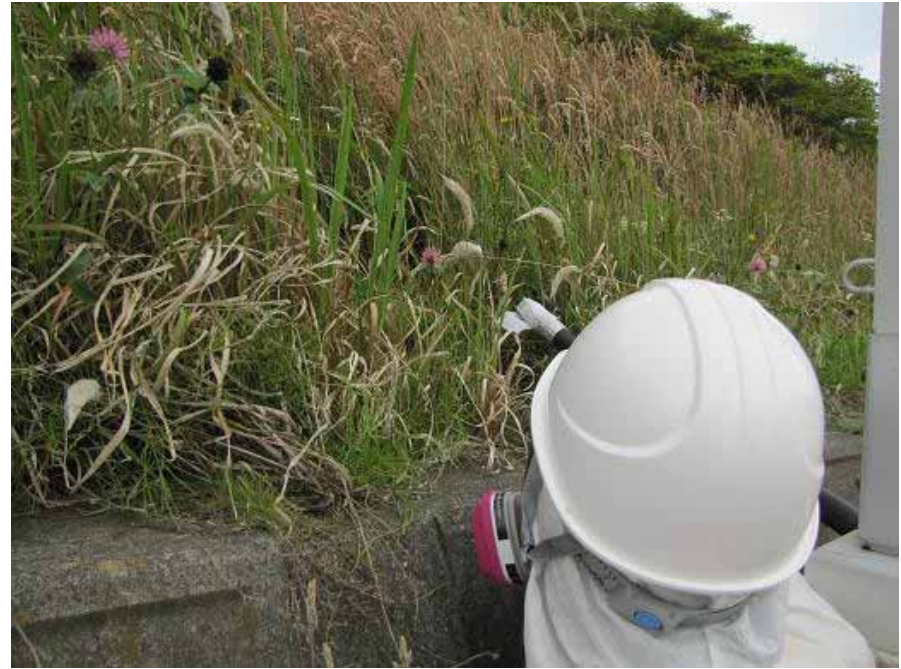
Temporary hose installation (Outside)
