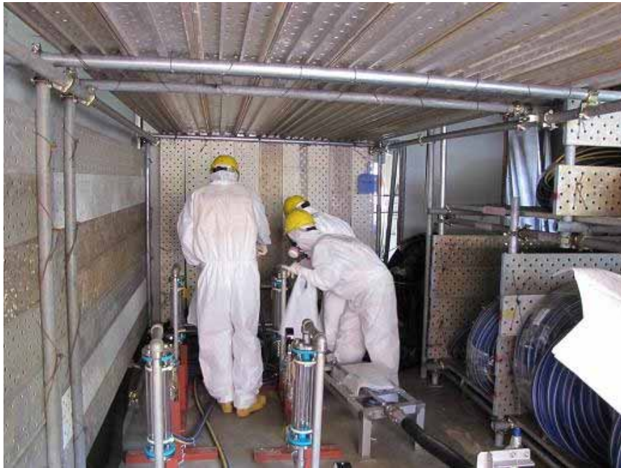
Temporary hose installation (in the Information Building)
