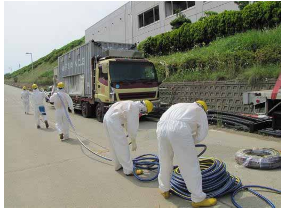
Temporary hose installation (Outside)
