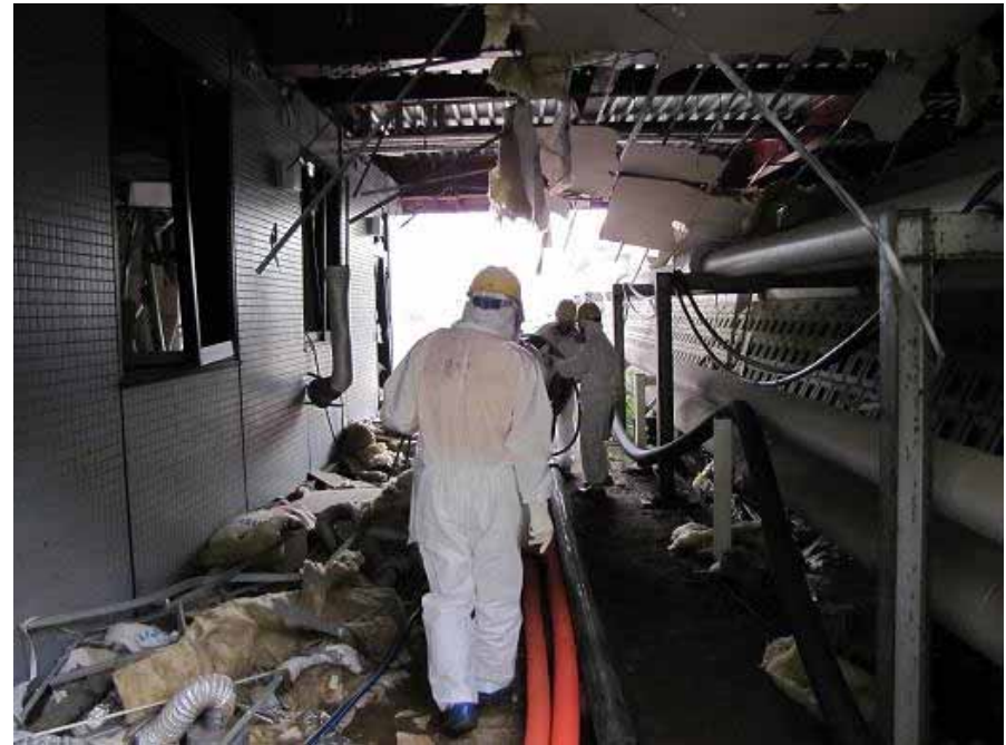
Temporary hose installation (in the Information Building)
