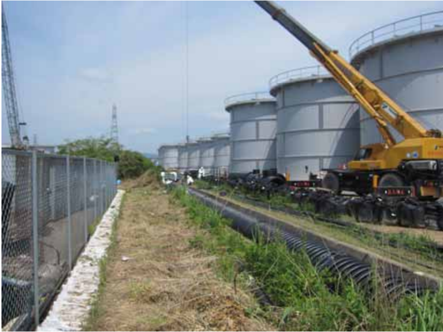
-1 PE pipe installation condition Photo taken by a TEPCO employee on June 18, 2012
