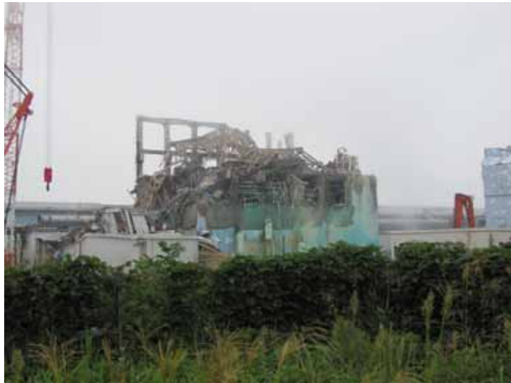
-1 Upper part of Unit 3 Reactor Building (Before debris removal) Photo taken by a TEPCO employee on September 15, 2011
