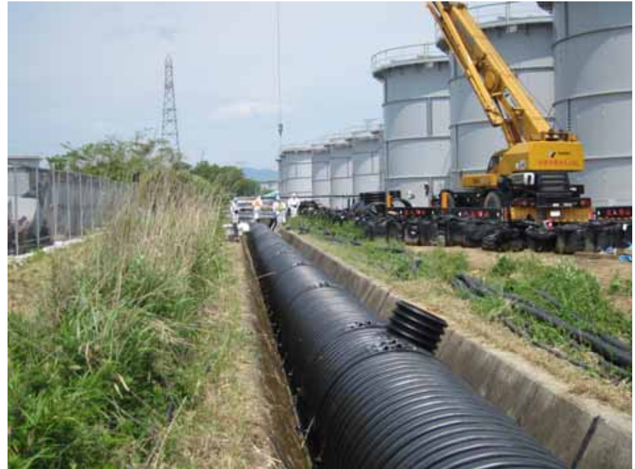
-2 PE pipe installation condition Photo taken by a TEPCO employee on June 18, 2012
