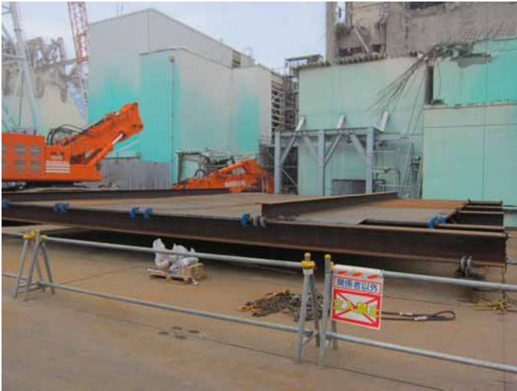
Unit 4 Spent Fuel Pool protection platform Photo taken by a TEPCO employee on June 7, 2012
