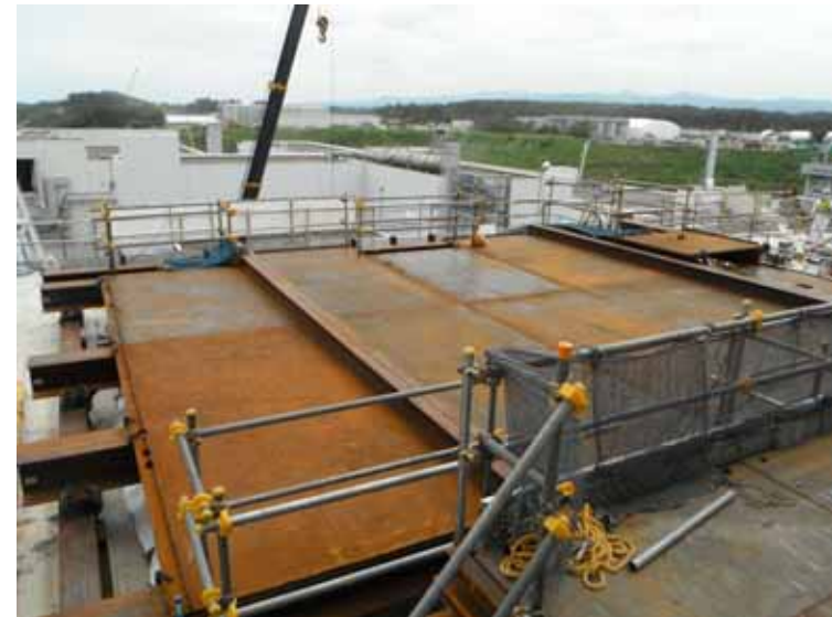
Platform installation completed (As announced on June 15, 2012)
