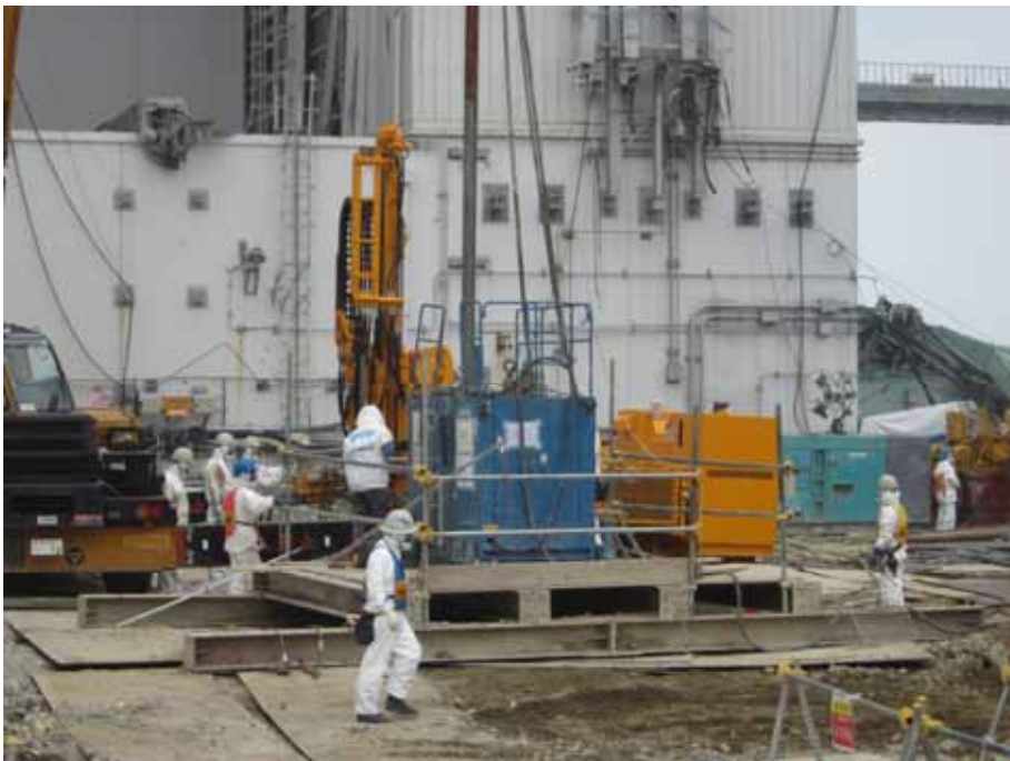
-1 Unit 4 south side foundation improvement work: Foundation improvement equipment Photo taken by a TEPCO employee on June 7, 2012
