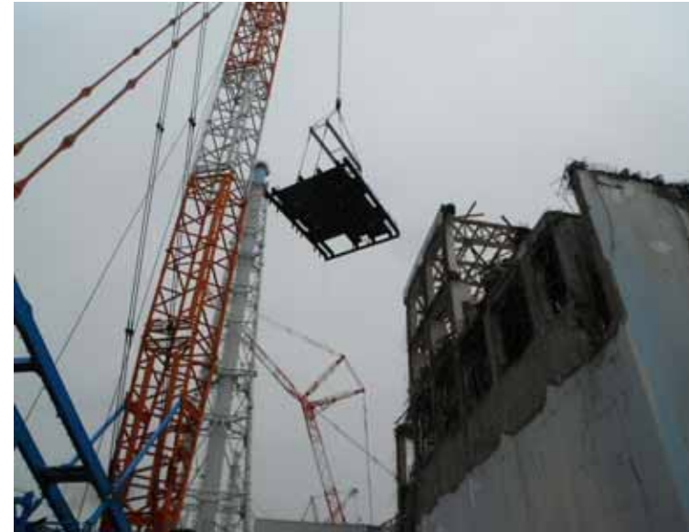
Lifting up the protection platform (As announced on June 15, 2012)
