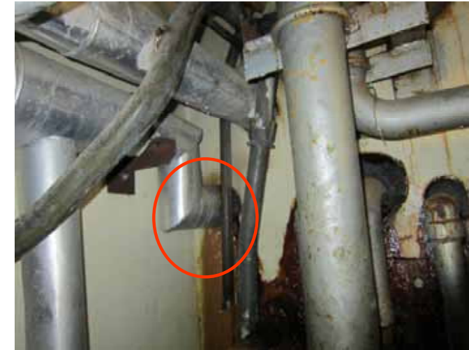
Location where water inflow was confirmed (Photo taken by a TEPCO employee on May 29)
