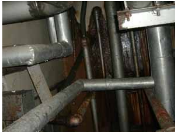
The location near where the water flow was confirmed
