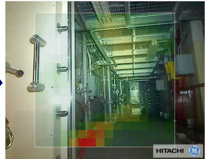
Processed data on the west aisle
