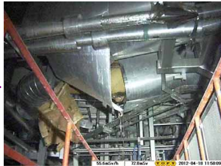
Upper part of the route of northeast
