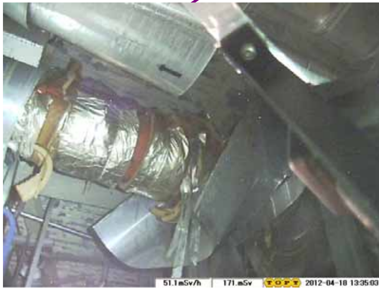
Upper part of the southeast S/C manhole
