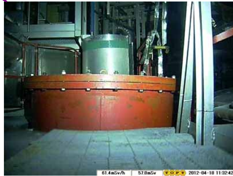
Southeast S/C manhole
