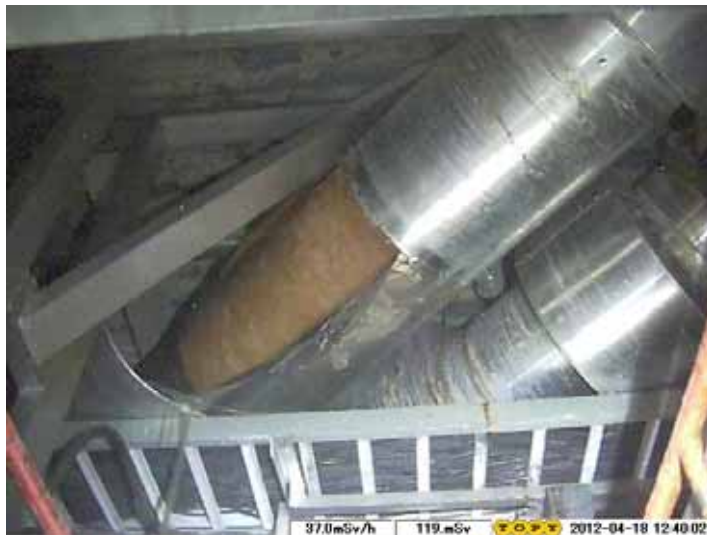
Upper part of the south route
