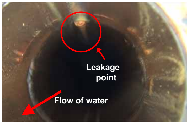
After valve removal (from upper part)
