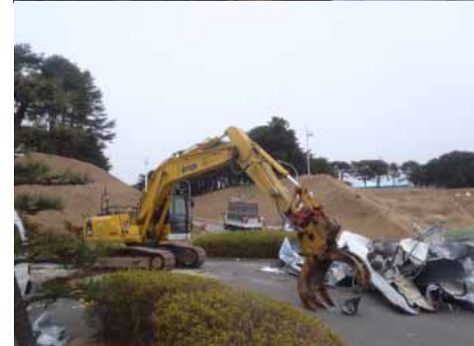
Removal of debris on the ground
