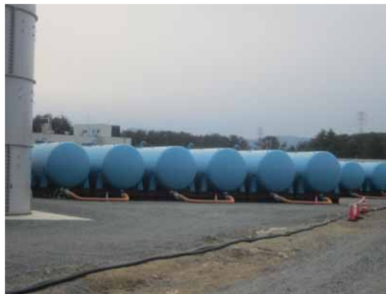
- 2 Tank array at H area Jan. 9, 2012 photo by TEPCO staff
