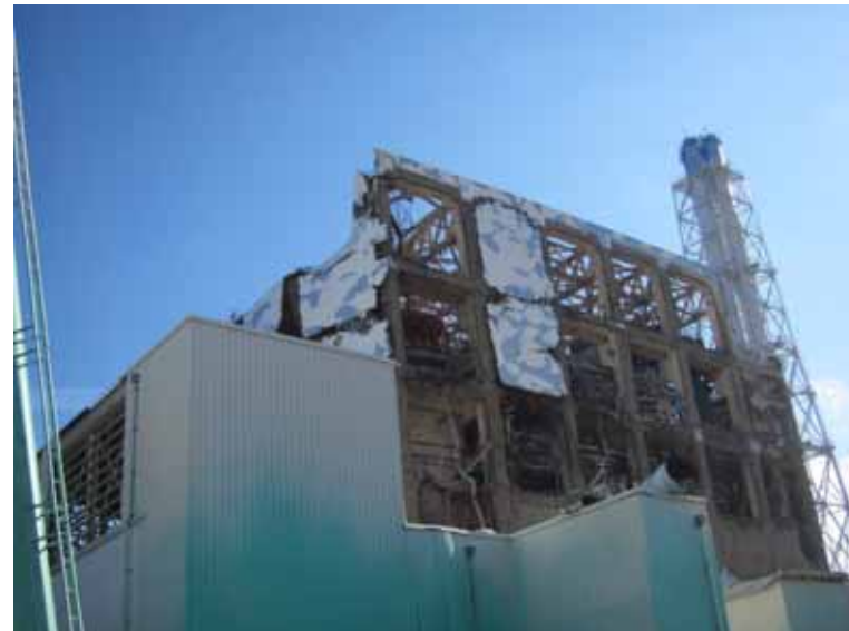
- 4 Unit 4 Reactor Building Jan.10, 2012 photo by TEPCO staff
