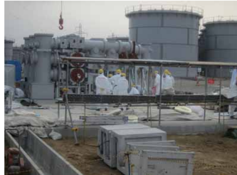
- 2 Construction of new switch station Jan. 9, 2011 photo by TEPCO staff
