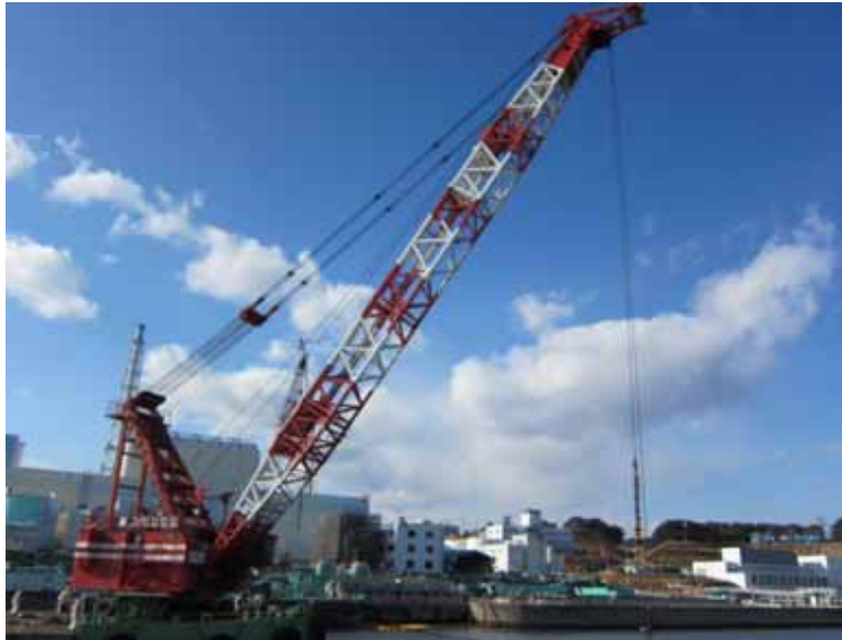
- 4 Removal of obstacle by the floating crane (from east breakwater)
