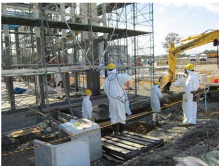
- 10 Construction of new switch station Jan.10, 2011 photo by TEPCO staff
