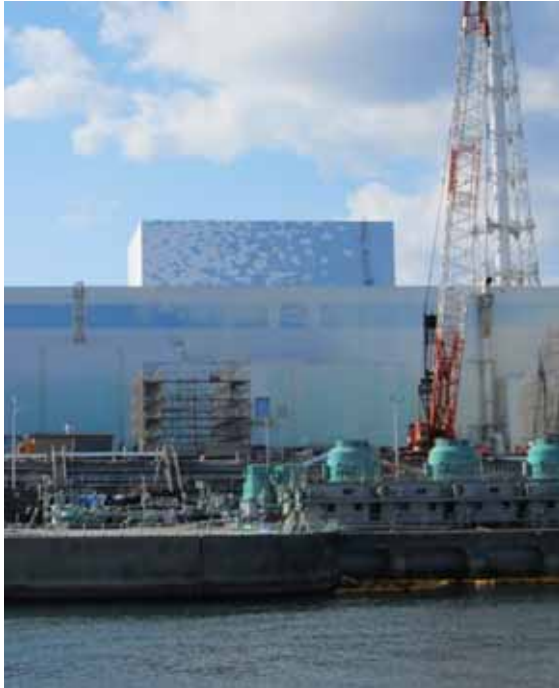
- 1 Unit 2 Turbine Building (from east breakwater)
