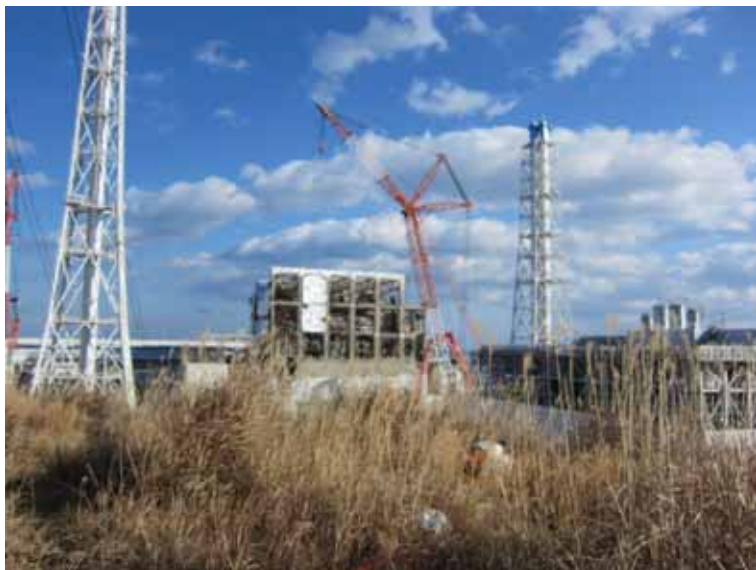
- 1 Unit 4 Reactor Building Jan. 14, 2012 photo by TEPCO staff
