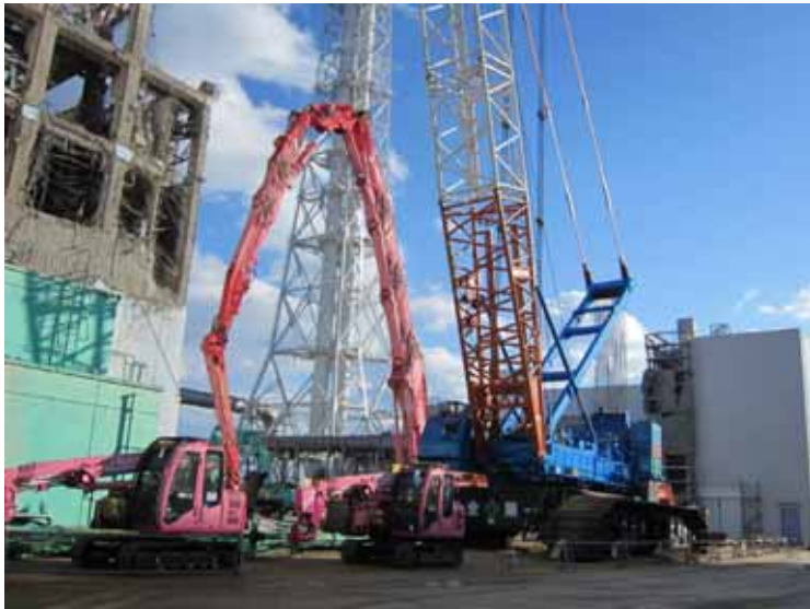
- 1 Large size heavy machine for dismantling Jan. 14, 2012 photo by TEPCO staff
