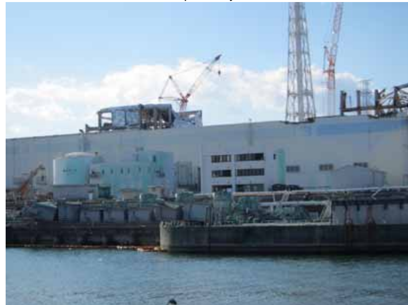
- 3 Unit 3,4 Turbine Building (from east breakwater)
