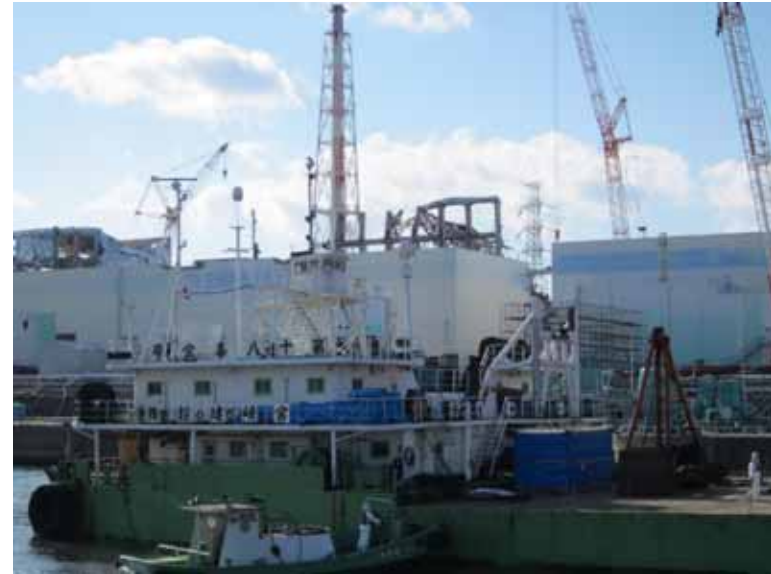
- 5 Removal of obstacle by the floating crane (from east breakwater)
