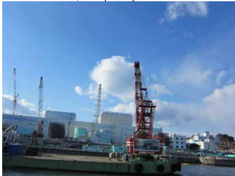
- 6 Removal of obstacle by the floating crane (from east breakwater)
