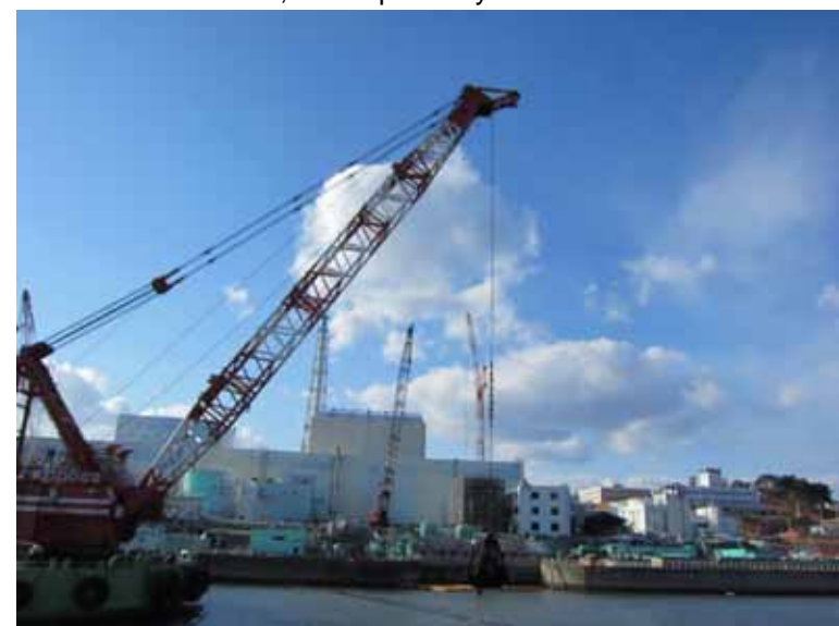
- 7 Removal of obstacle by the floating crane (from east breakwater)
