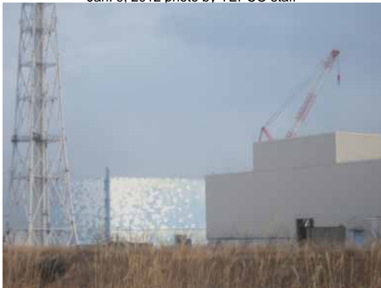
- 3 Look into Unit 1 Reactor Building from the backside of Main Anti-earthquake Building
