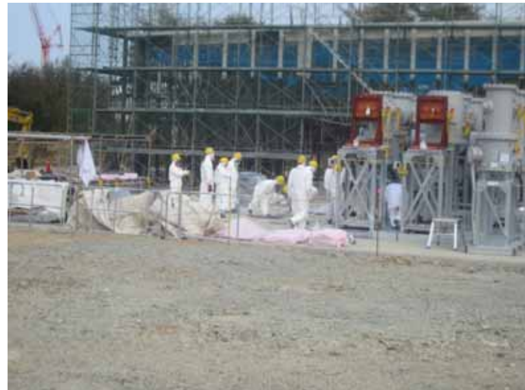
- 4 Construction of new switch station Jan. 9, 2011 photo by TEPCO staff
