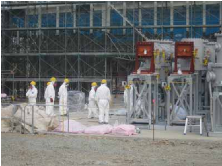
- 5 Construction of new switch station Jan. 9, 2011 photo by TEPCO staff
