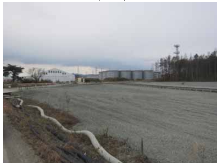
- 3 Look into west side from the hill in the southern side of Unit 4 Jan. 9, 2012 photo by TEPCO staff
