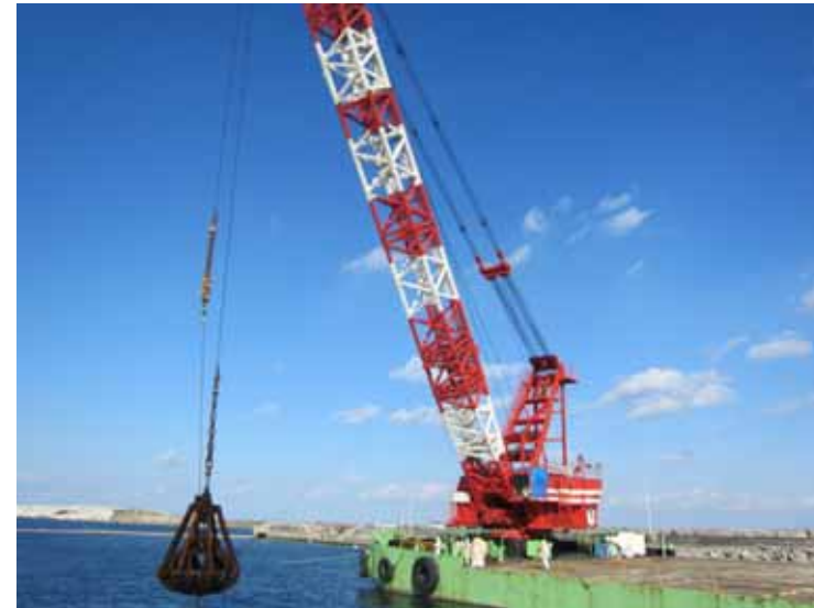
Removal of obstacle by the floating crane (from sea side yard)
