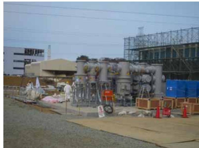
- 7 Construction of new switch station Jan. 9, 2011 photo by TEPCO staff
