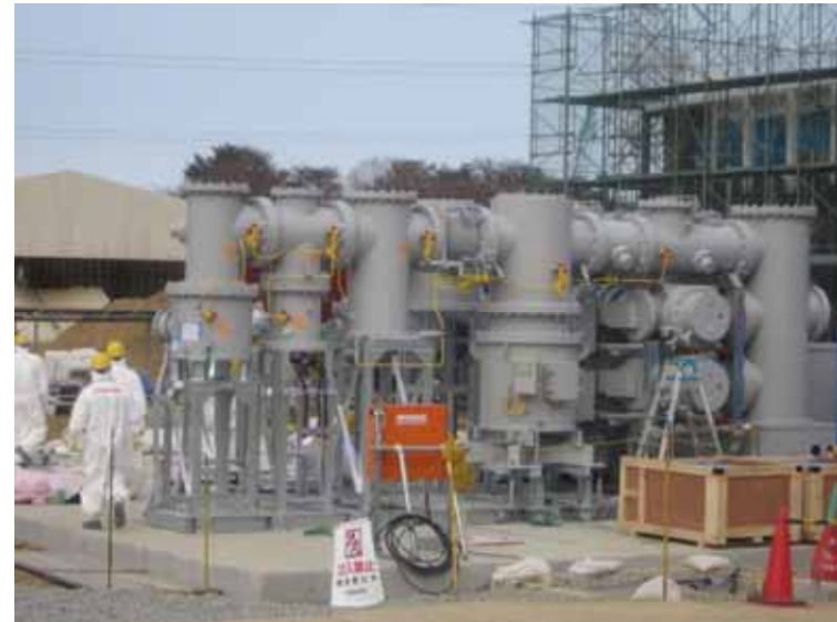
- 6 Construction of new switch station Jan. 9, 2011 photo by TEPCO staff
