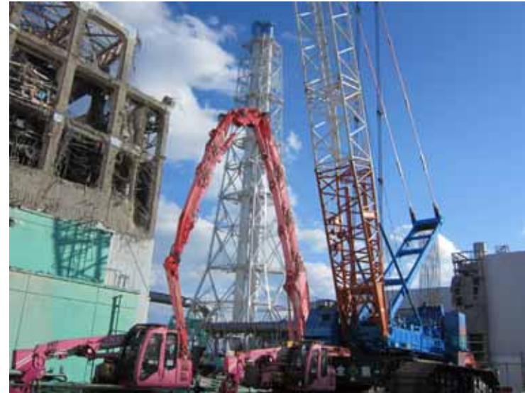
- 2 Large size heavy machine for dismantling Jan. 14, 2012 photo by TEPCO staff
