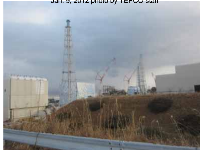
- 4 Look into Unit 1 Reactor Building from the backside of Main Anti-earthquake Building
