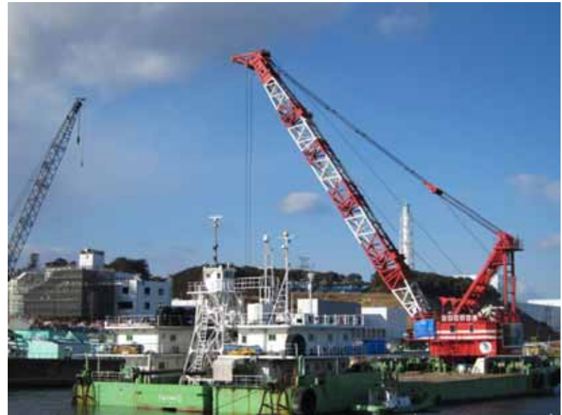
- 2 Removal of obstacle by the floating crane (from east breakwater)
