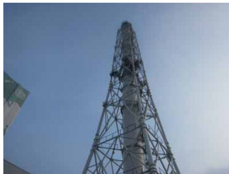
Unit 5,6 Stack Jan. 9, 2012 photo by TEPCO staff
