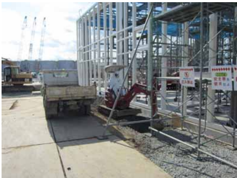
- 8 Construction of new switch station Jan.10, 2011 photo by TEPCO staff
