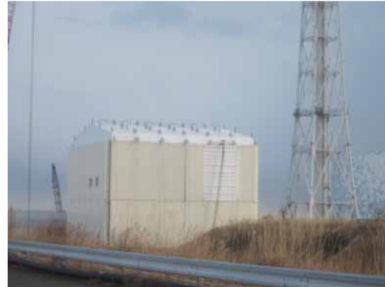
- 2 Look into Unit 1 Reactor Building from the backside of Main Anti-earthquake Building
