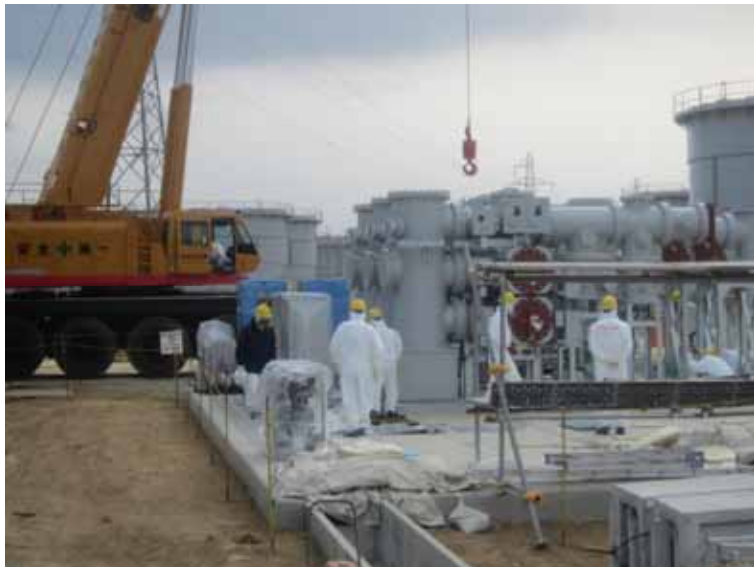
- 3 Construction of new switch station Jan. 9, 2011 photo by TEPCO staff
