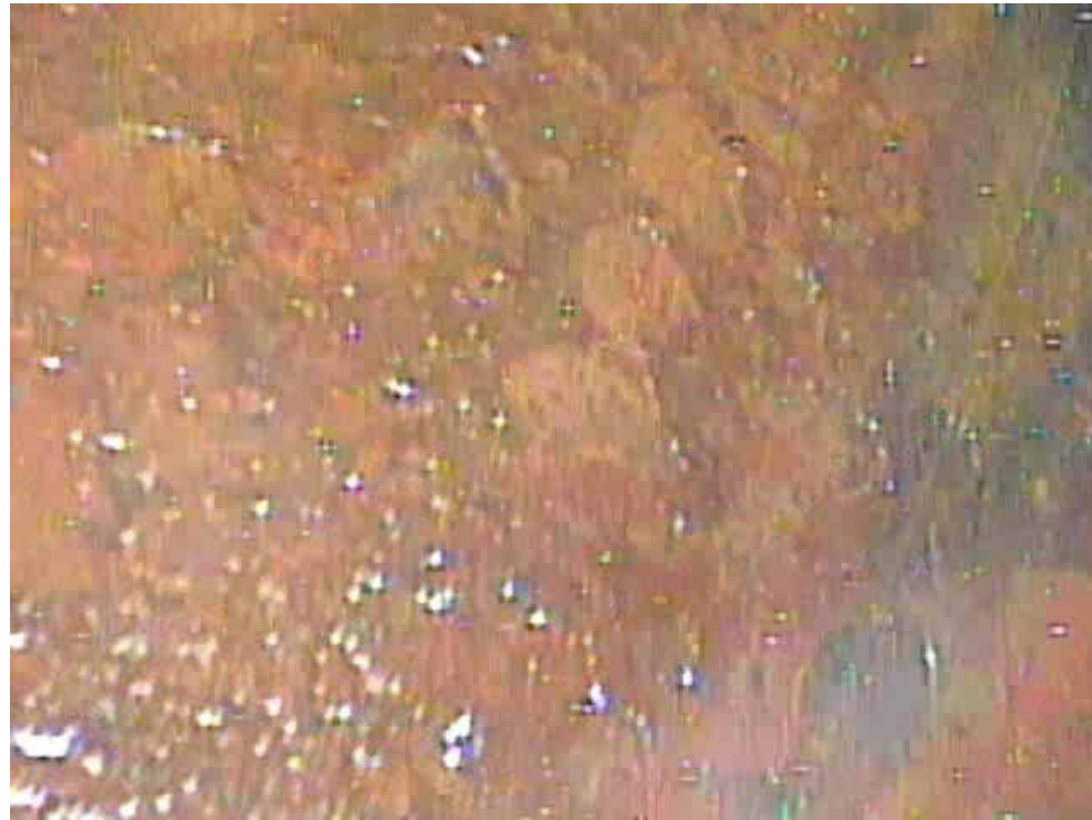
Internal wall of PCV
