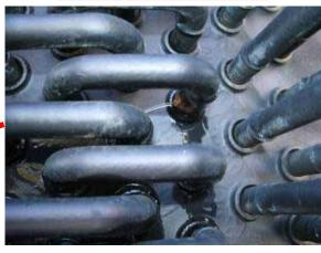
Air Fin Cooler B2: 2 points leakage Air Fin Cooler B3: 2 points leakage
