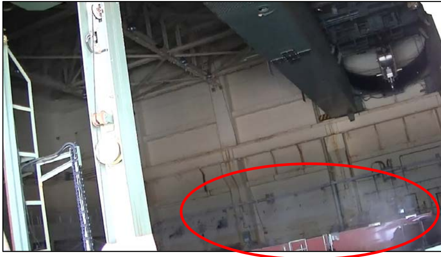
Condition of the directly above the reactor at 5 th floor : Generated steam (photo taken on Sep. 17)
