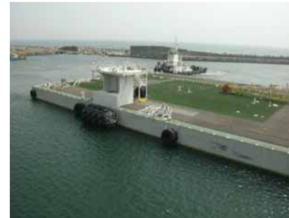
Tank for low concentrated accumulated water (Mega float)
