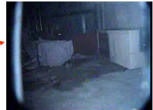
In Front of the Equipment Hatch at North-East Area
