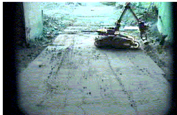
Under the Equipment Hatch at South-West Area
