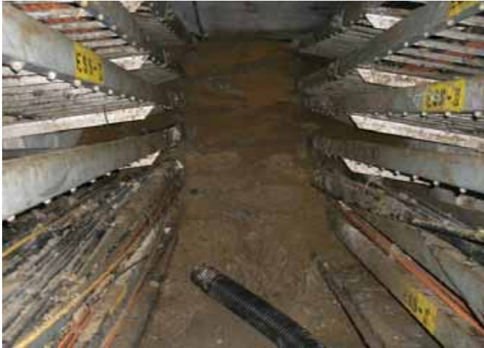
( 29 ) Unit 5 Water intake cable pit Taken by TEPCO employee on August 25,2011
