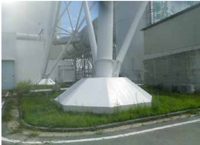
( 31 ) Unit 5 Basement of Main exhaust stack Taken by TEPCO employee on September 7,2011
