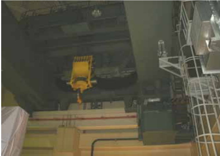
(21) Unit 6 Reactor building ceiling crane Taken by TEPCO employee on August 24, 2011
