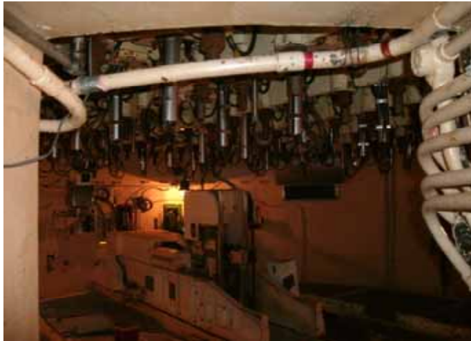
(5) Inside Unit 5 pedestal (reactor foundation) Taken by TEPCO employee on August 17, 2011
