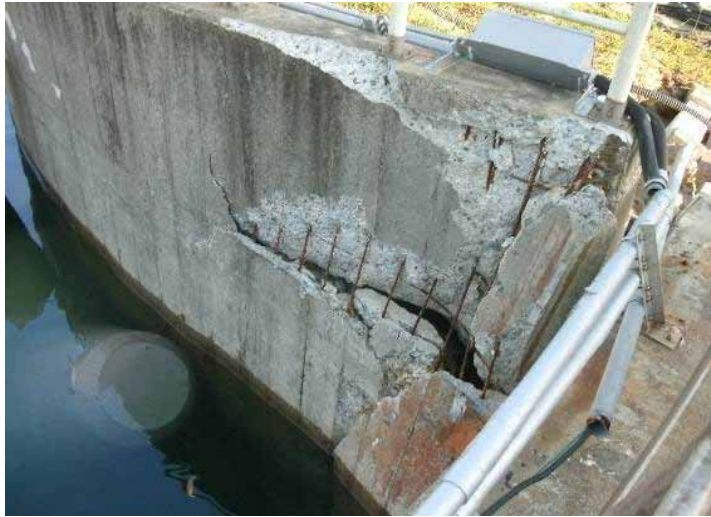
( 25 ) Unit 5 Intake channel Taken by TEPCO employee on August 23,2011
