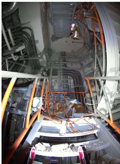
Staircase from 2nd floor to 3rd floor
