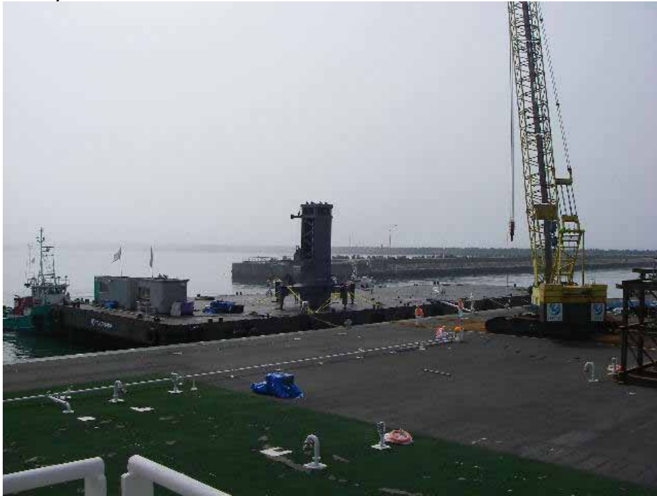
Photo: Tokyo Electric Power Company
