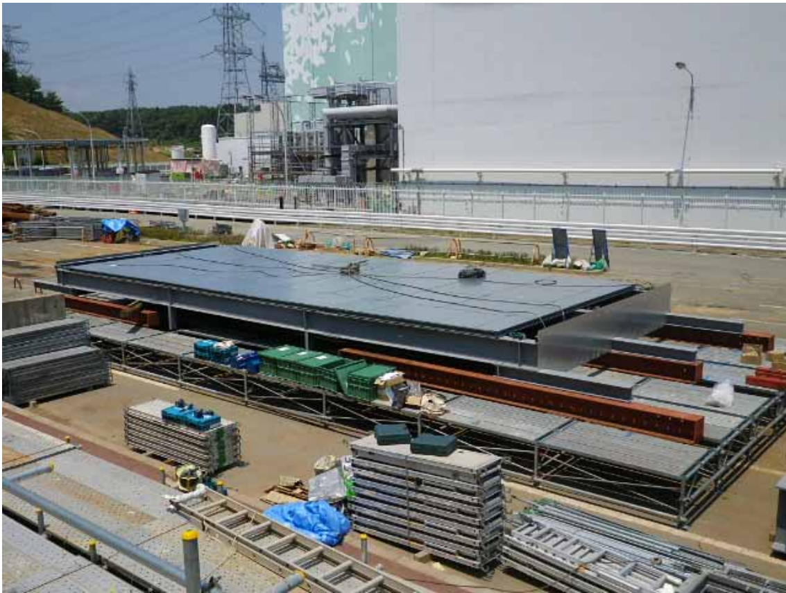
Appearance of the Roof for Countermeasure against Rainwater, Unit 3, Fukushima Daiichi
