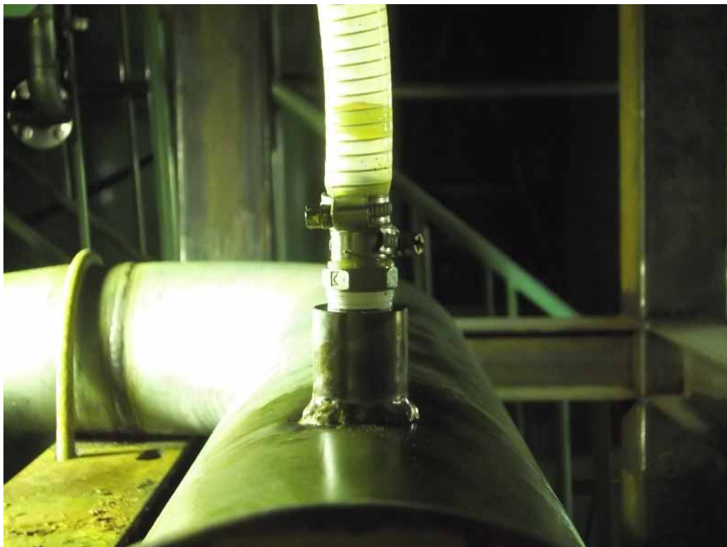
Hose Connection (after repair)
