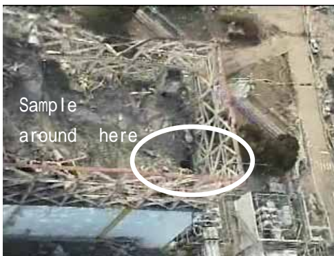
Unit 1 (north west corner)
