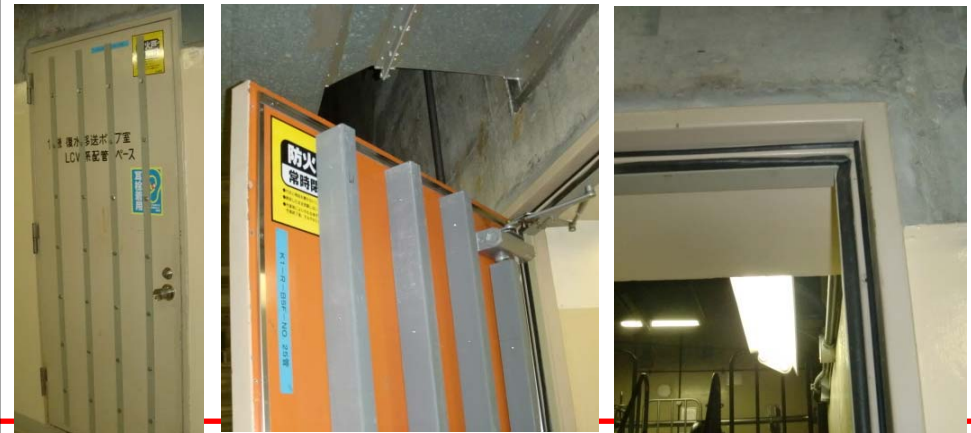
Reinforcement Steel Installation
