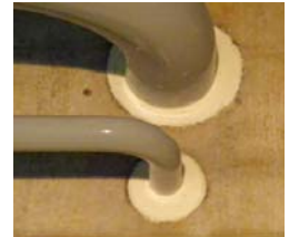
Waterproofing Building Hole
