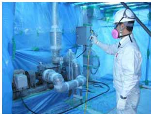
Spraying the dust inhibitor
