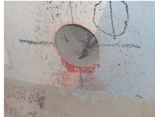
Core drilling point for core sampling
