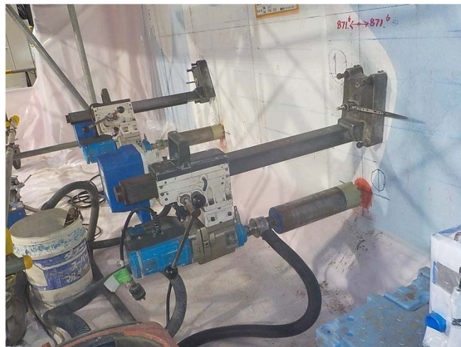
Installation of core drilling machine Photo taken on April 16, 2018
