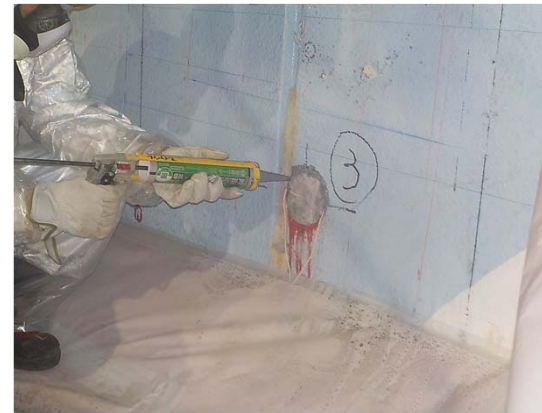
Filing in drilled core hole
