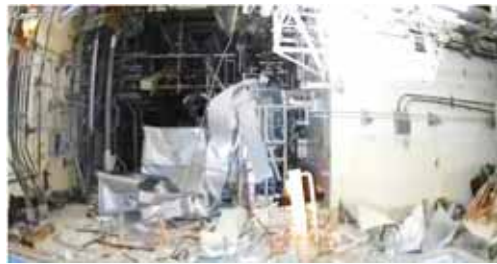
Photo③ North from 2 nd floor opening
