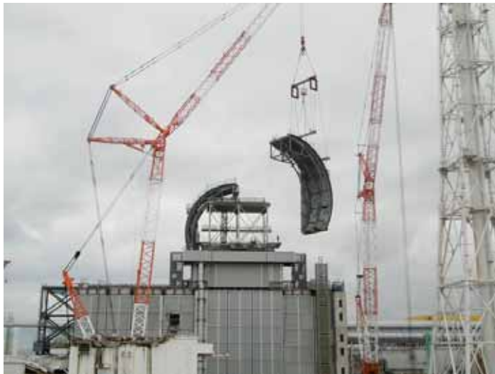
Lifting up dome roof
