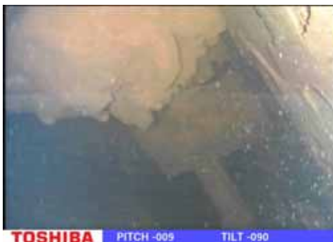
⑧ Nearby the wall of pedestal
