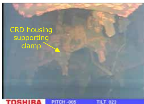
Bottom of the CRD housing
