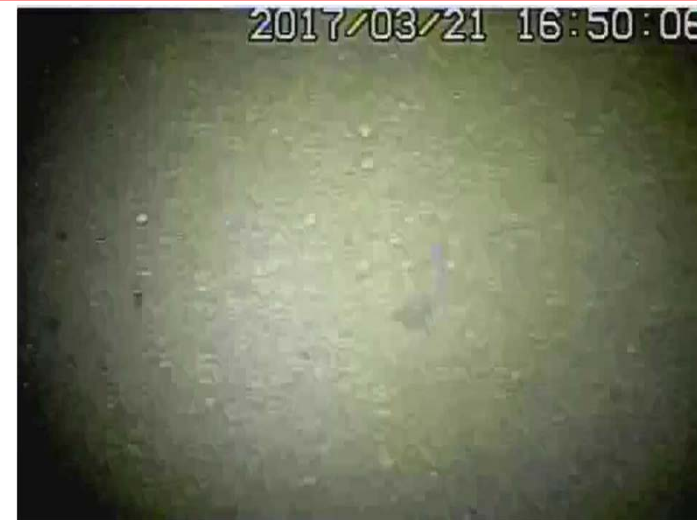
Underwater image between the measurement points D1 and D2
