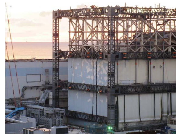
After removal of the panel
