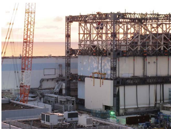
Before lifting up the panel
