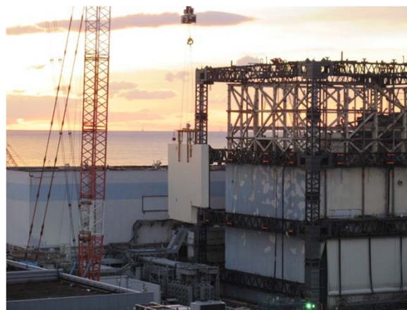
Lifting up the panel
