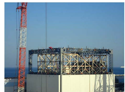
After removal of the panel
