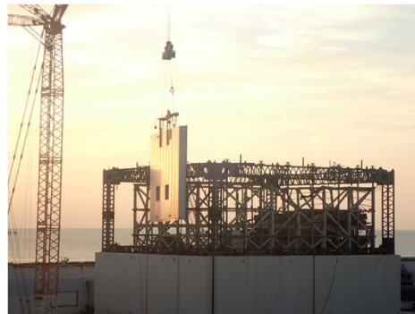
Lifting up the panel
