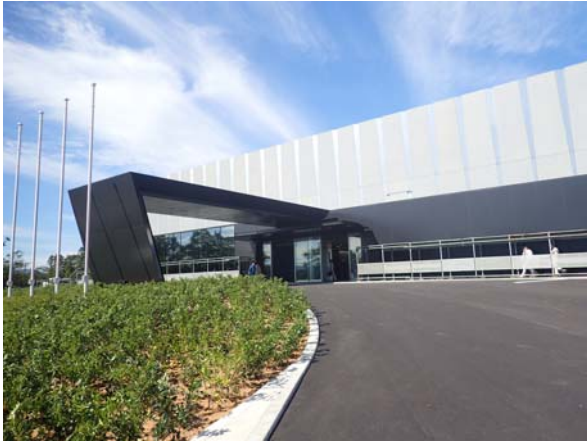
Exterior of new administration building
