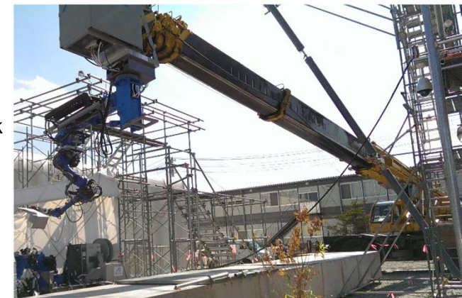
Mock-up tests using remotely controlled robots
