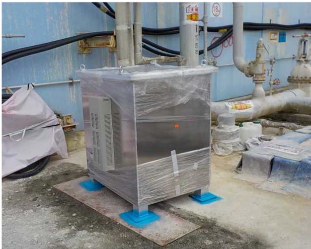
Installation of muon-measuring device (downsized to approx. 1m × 1m × 1.3m(height))
