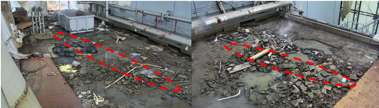
Before Cleaning Up Rubble on the Small Attached Annex
