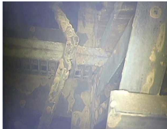
2. X-6 penetration and CRD rail
