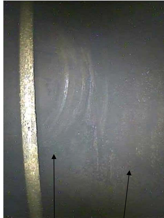
RHR pipe and PCV' inner wall
