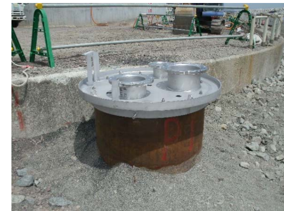
Groundwater drain pit (in front of the Unit 1 intake)
