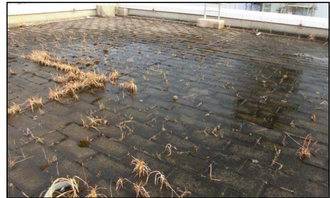
Photo④ : large carry-in entrance rooftop
