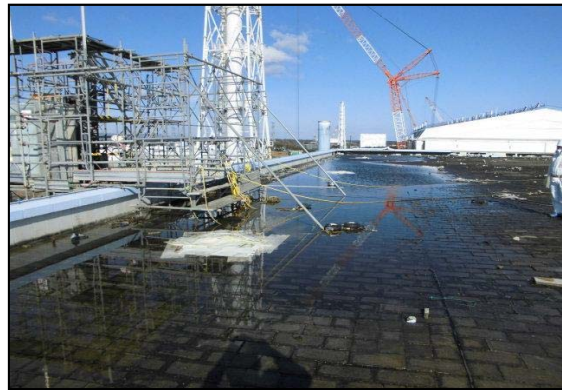
Photo② : Unit 2 Reactor Building rooftop
