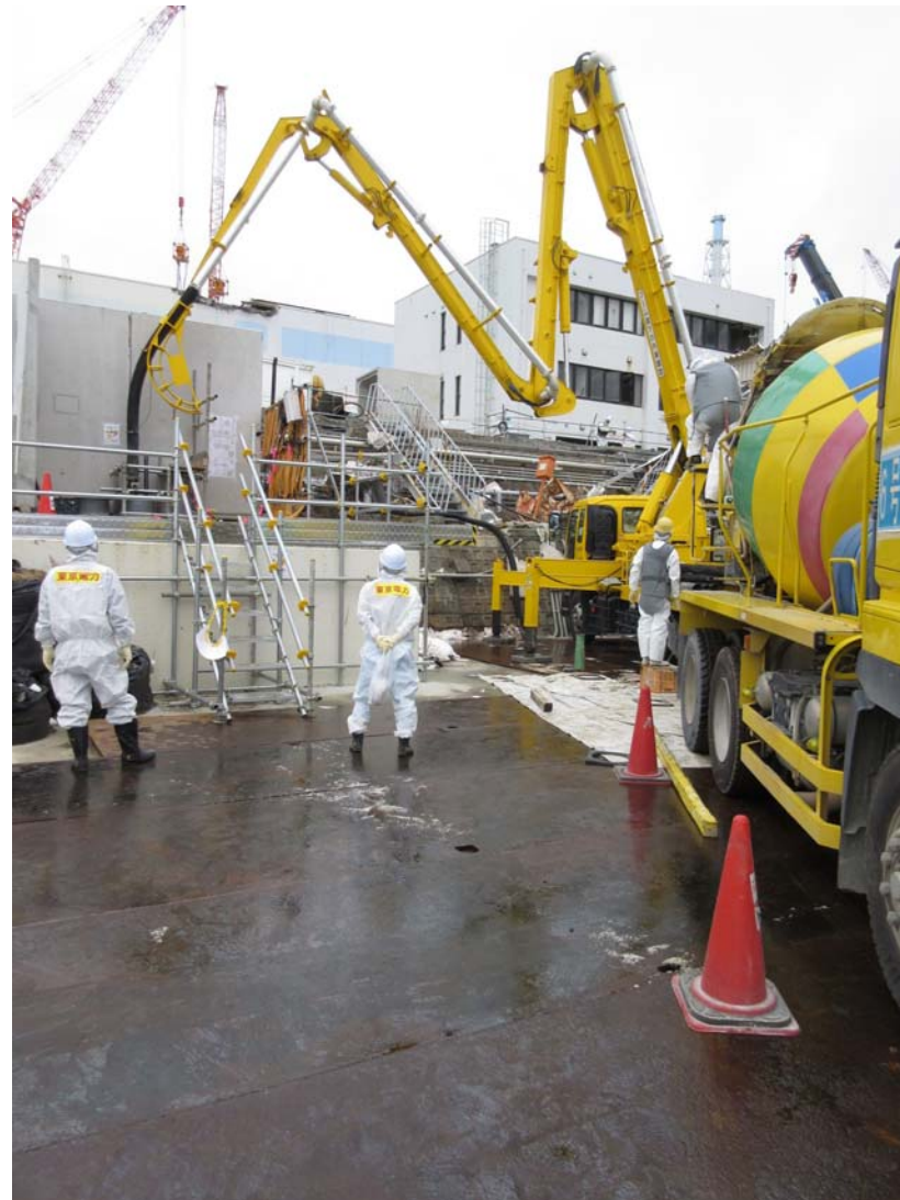
Filling of seawater pipe trench
