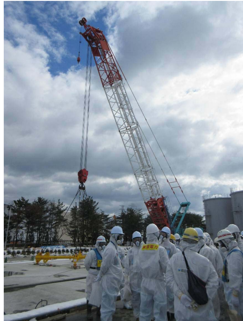
Meeting for K2 Tank area base construction before recommencement 3 rd February,2015
