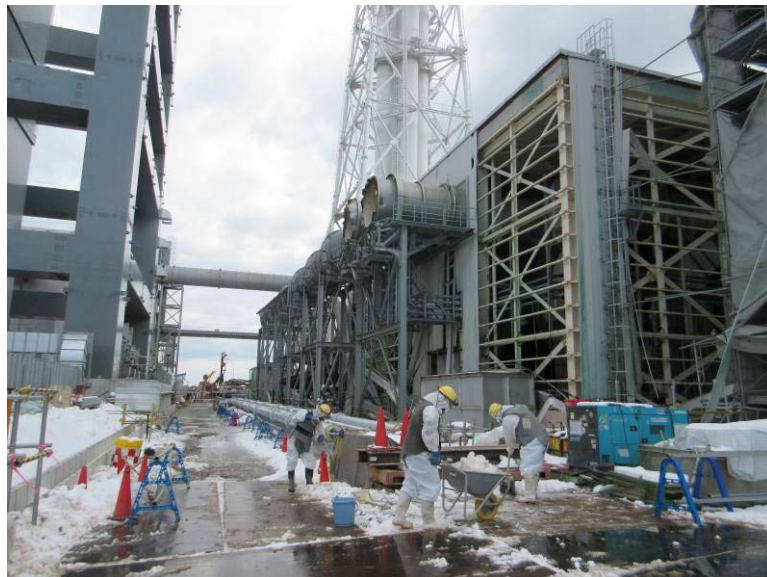
Landside impermeable wall construction
