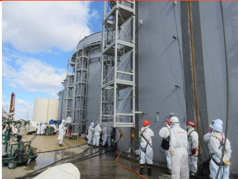
Safety confirmation around the J4 Tank area
