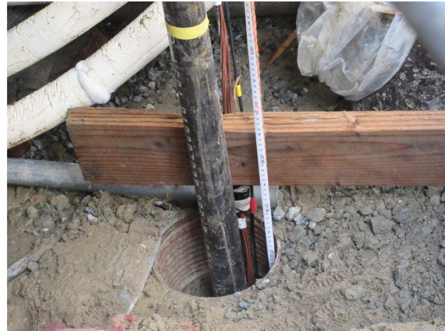
Around the filling pit
