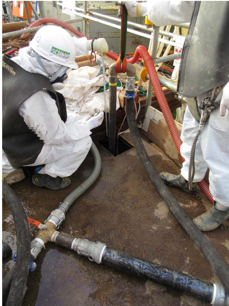
Seawater piping trench of Unit 2: Gap-filling operation of drilling duct
