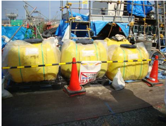
No sign on tanks put temporarily
