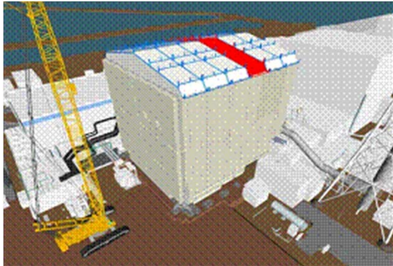
1) Roof panel dismantling start
