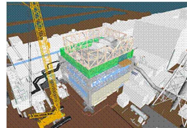
6) Cover dismantling completed Followed by debris removal
